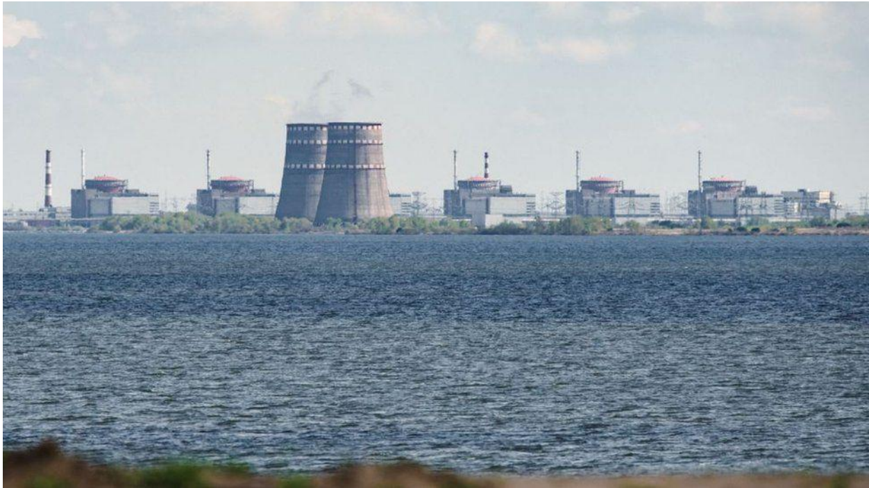
The six reactors (one partially hidden) and two cooling towers of the Zaporizhzhia nuclear plant.
